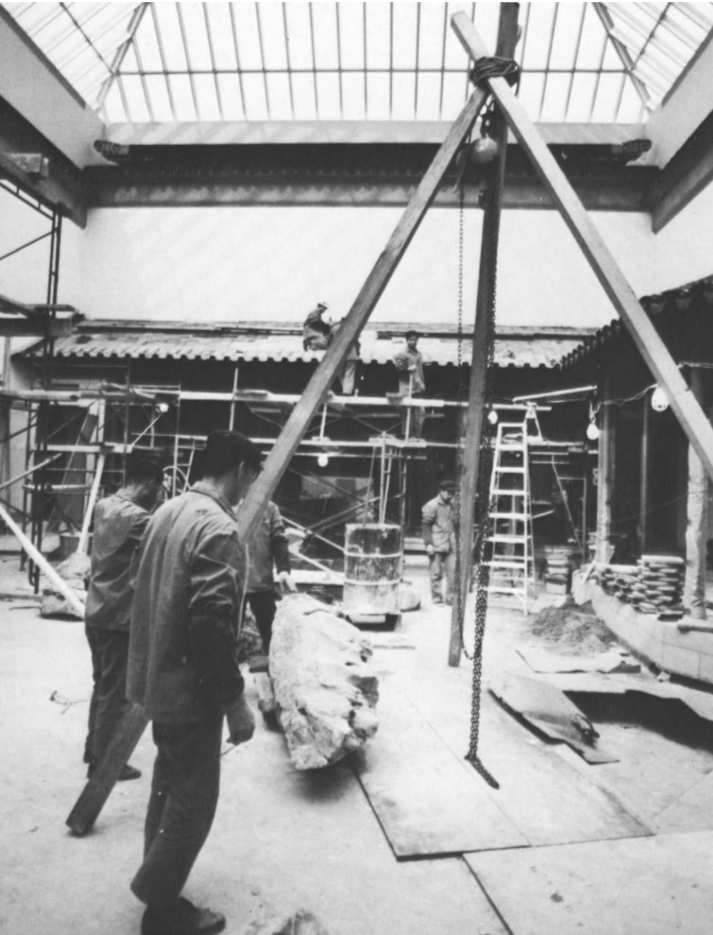
54. Using a traditional tripod, Chinese workmen maneuvered the large Taihu rocks into place. "Artificial mountains" were arranged along the walls as well as in small planters such as this one.
