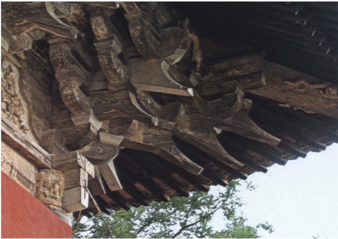
Figure 89. Corner-bracket set. Sanqingdian, Yonglegong, Shanxi Province
