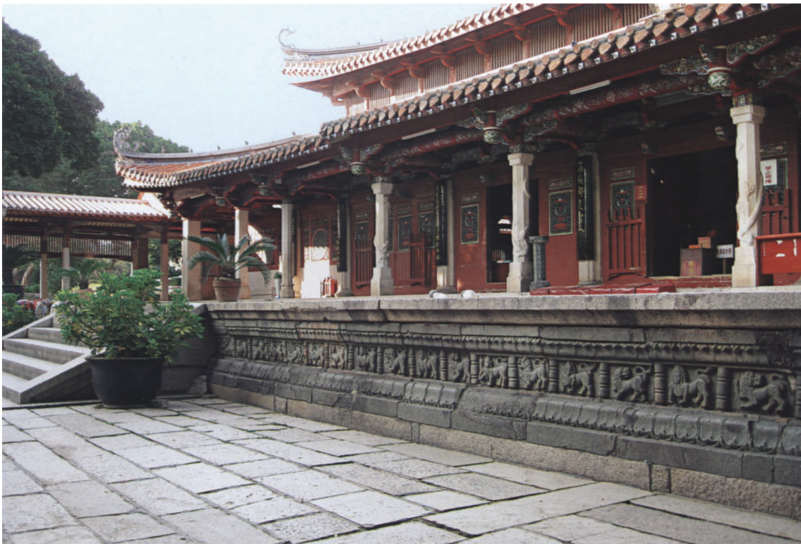
Figure 189. View from the southeast of the main entrance to Great Treasure Hall (Daxiong Baodian), Kaiyuansi, Quanzhou, Fujian Province, 2009. The foundation platform is inset with diorite greenstone panels and moldings in a South Indian Chola style depicting Hindu mythical creatures and lions between lotus-petal friezes.
